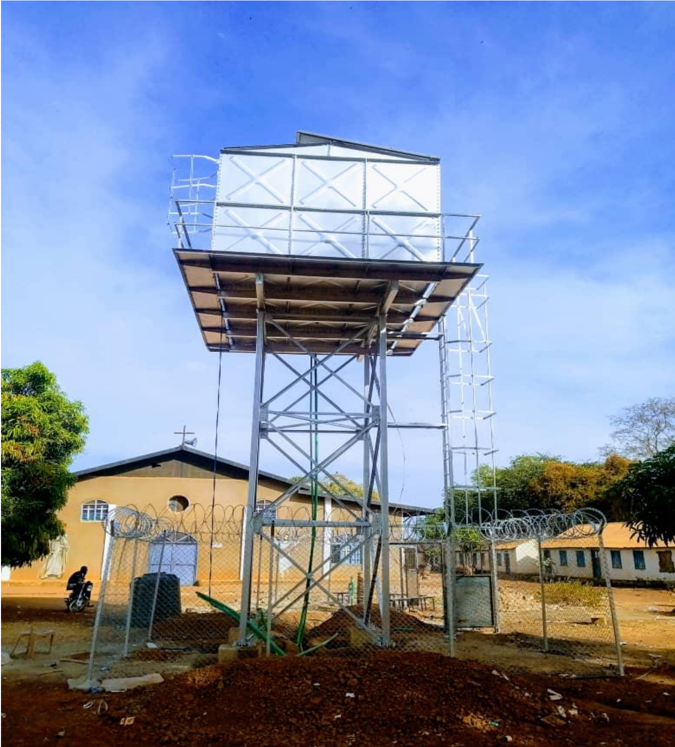
Figure 6: Water Tank and the fence with security wires 28/12/2025.
