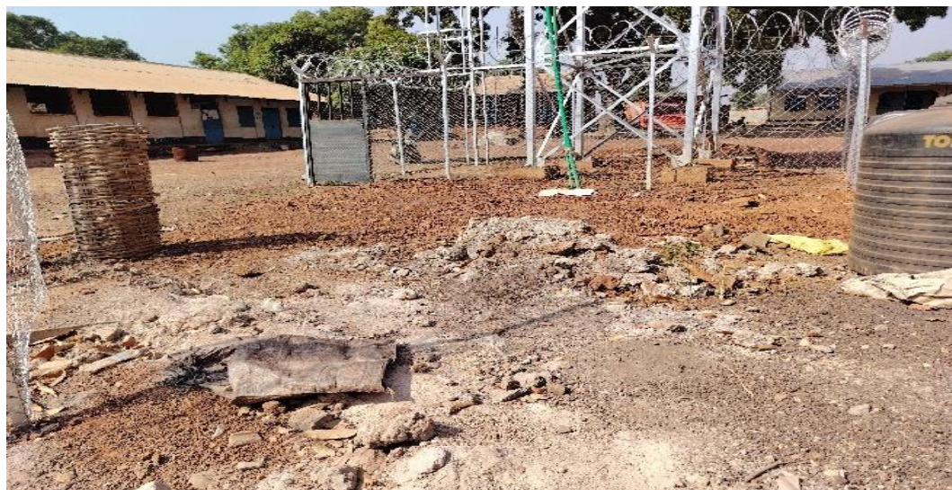
Figure 12: Indispose excess soil
